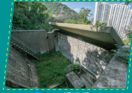
F 泥石壩 Check Dams
