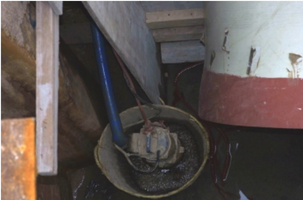
Plate B6 – Pumping provided
